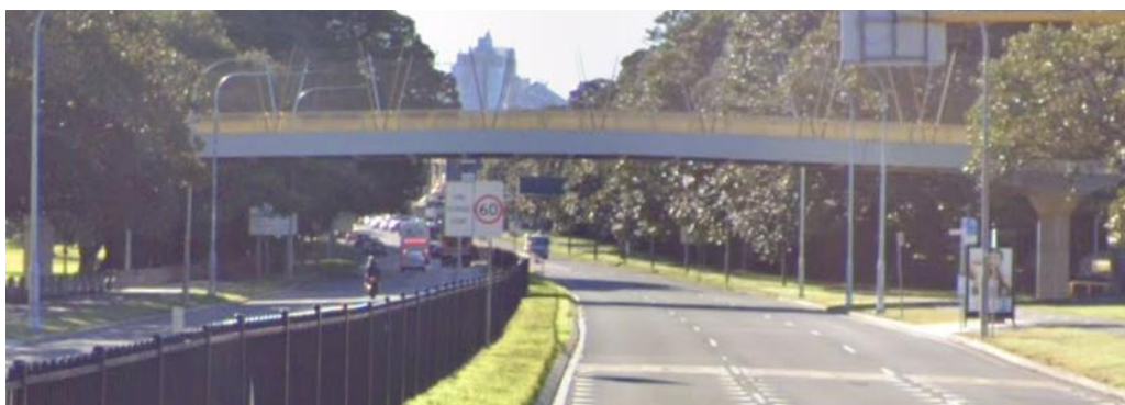
Albert ‘Tibby’ Cotter Footbridge at Anzac Pde
