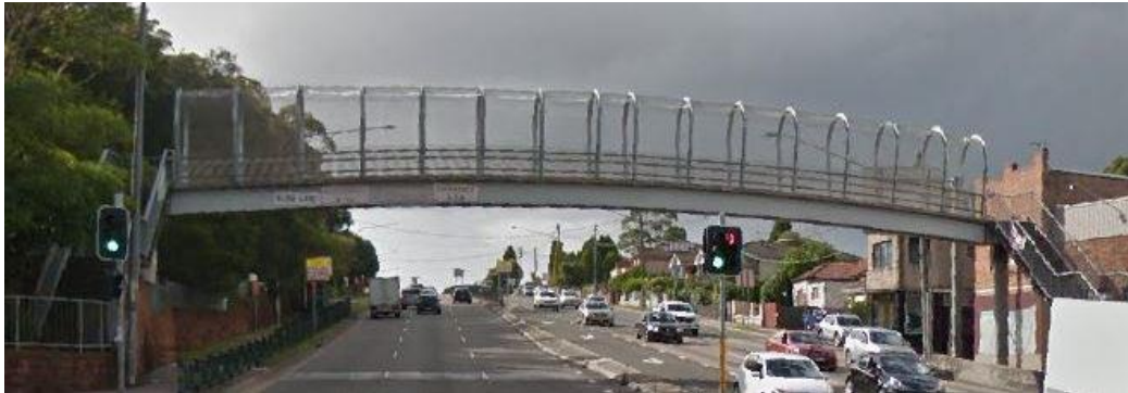
King George Road Footbridge, Beverly Hills
